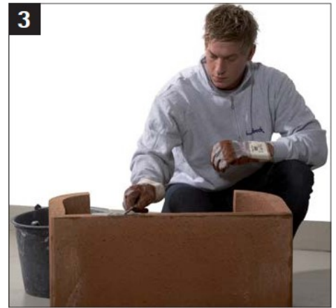
3 Apply mortar on the lower edge of the base and wood storage
