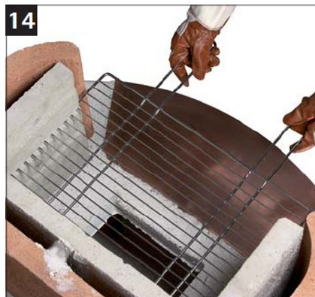
14 Use the chrome cooking grill to measure the correct distance between the firebox side panels.
