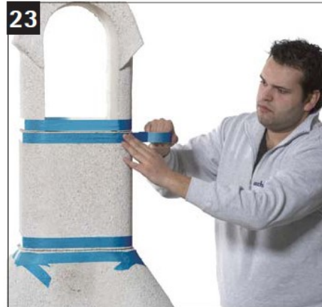
23 For a neater, finished look, use masking tape above and below the seams.
