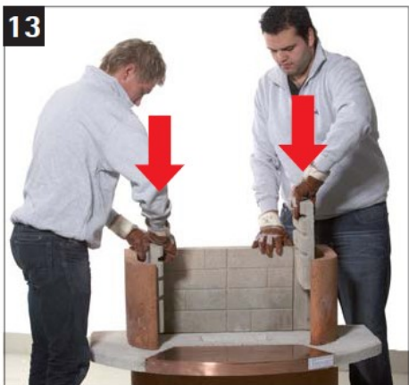
13 Place the side firebox components with the bevel at the front and the grill support slots at the higher levels. Make sure side panels are straight and parallel with each other.
