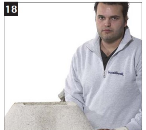
18 Apply mortar on the upper edge of the concrete hood
