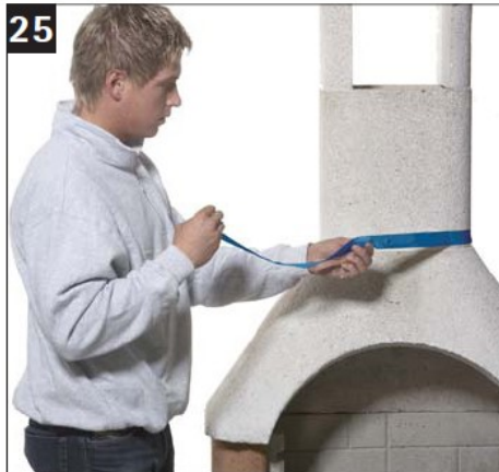
25 Remove the tape after the mortar sets.
